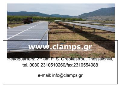
After many years of experience in fixed as well as mobile photovoltaic mounting systems, our company has created the new single axis (East-West) TRACKER SSH 5000 model.
